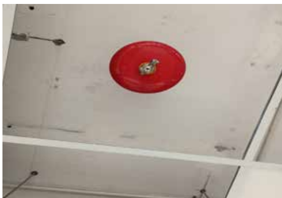
Zero ODP Modular Fire Suppression System
