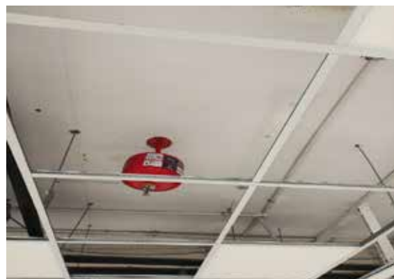
Zero ODP Modular Fire Suppression System
