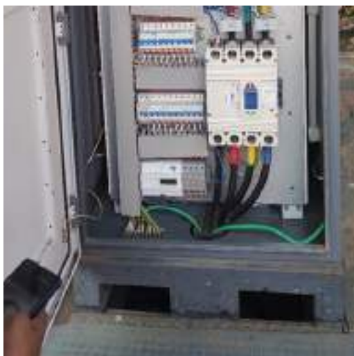
Missing phase separator Improper glanding and wrong colour code
