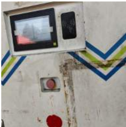
No identification label for Emergency PB
